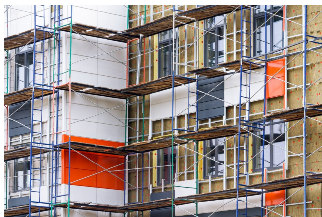
Mineral wool is used as thermal insulation in buildings. With our knowledge in regulations, DHI has prepared a comprehensive REACH registration dossier for mineral wool. © Shutterstock / Mr Twister
